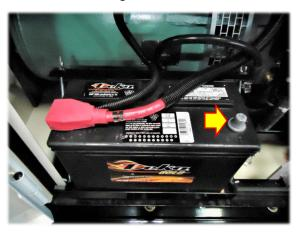
On the backside of the lug panel, remove and retain the nut, lock washer and flat washer from the ground lug stud
