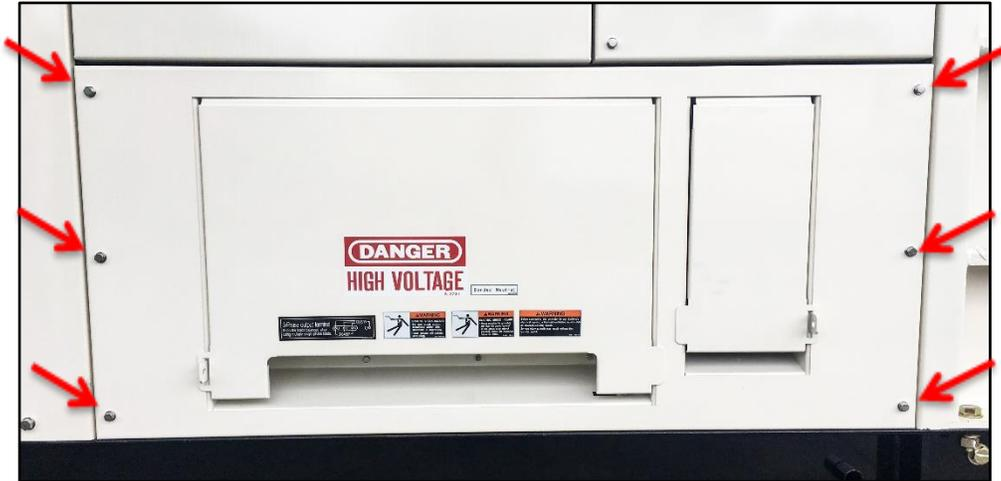
12. Confirm the decals are applied on the control panel and on the output terminal panel
