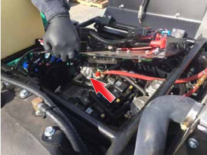
Figure 14. Lift Electrical Panel
