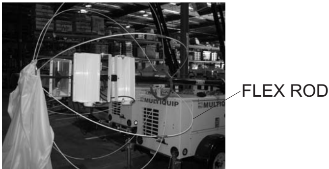
Figure 10. All Flex Rods Installed
