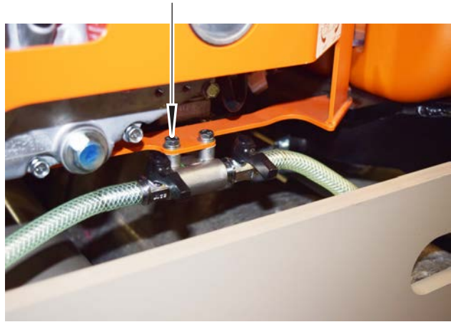
Figure 10. Removal of T-Connector Bolts
