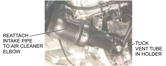
Figure 16. Reconnecting Intake Pipe
