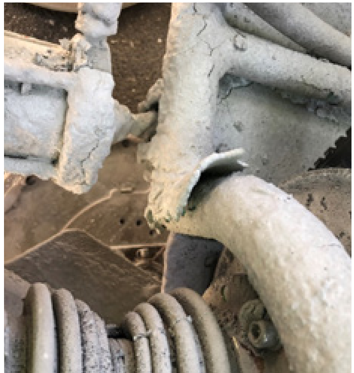
Slurry build up on frame and steering cylinder.
