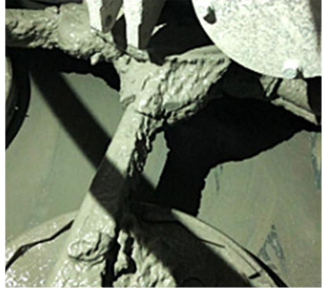
Heavy slurry build-up on arms and pitch bolt area also add weight to the unit. When rotating this makes for an out of balanced rotation resulting in damaging vibrations.
