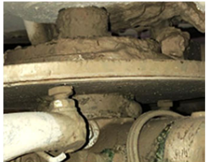
Heavy slurry built up on the spider and thrust plate area. Bearing and bushing failure will occur as well as potential for the gearbox output shaft seal to be damaged.
