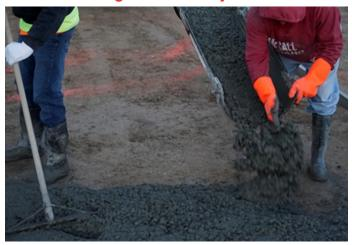
When cement is mixed with water a reaction occurs known as *hydration*.
