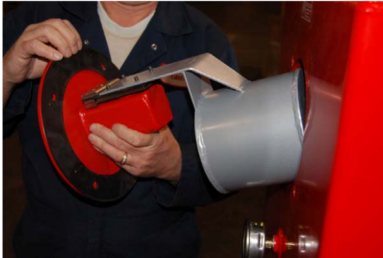
Figure 2. New Float Valve and Gasket Installation
