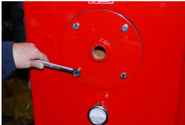
Figure 1. Float Valve Removal
